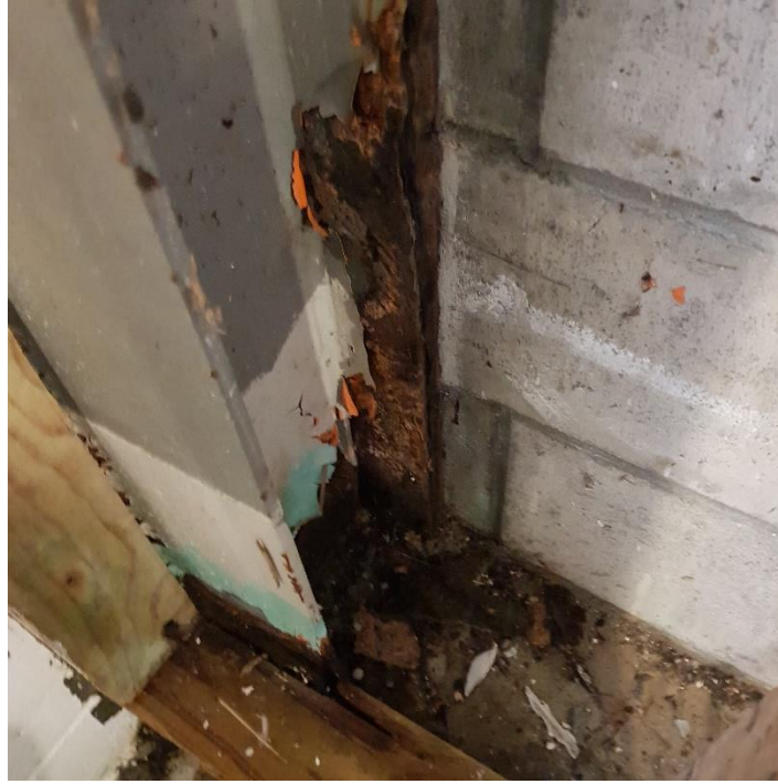
Severe corrosion of steel column flanges and base plate
