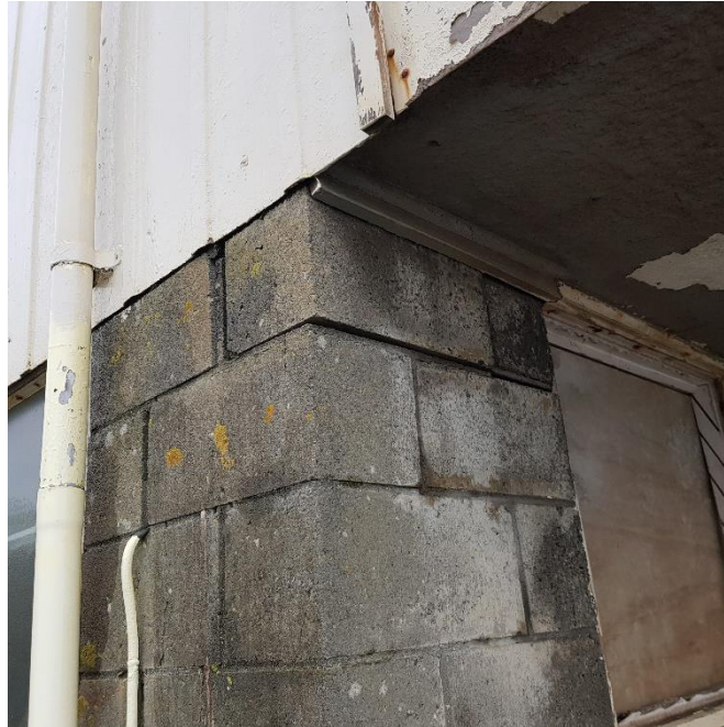
Loose blocks in northwest wall corner
