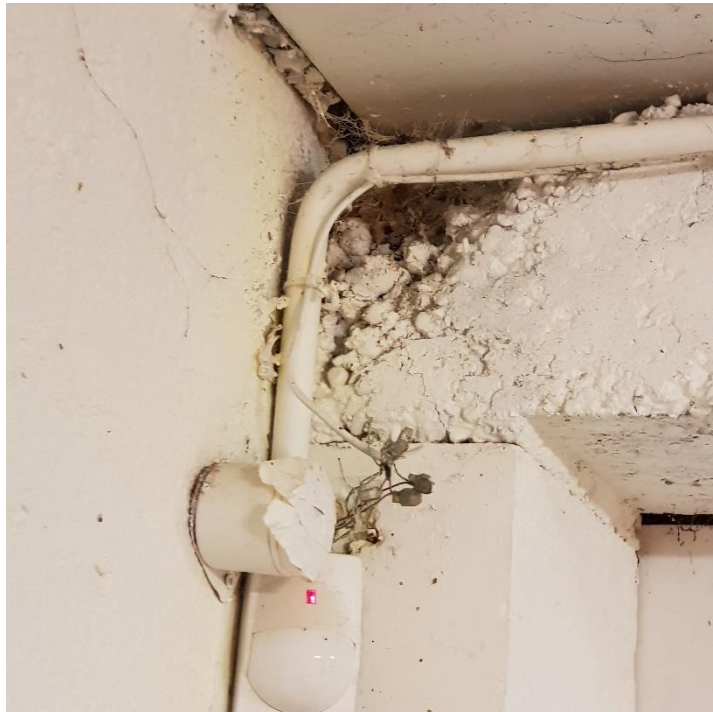
Honeycombing of concrete in critical beam/column joint
