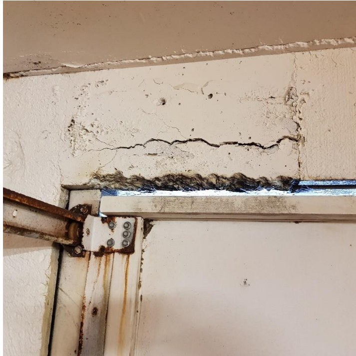
Cracking in concrete floor beam
